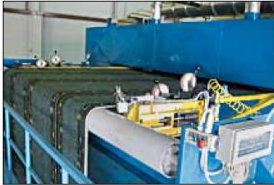
Stenter inlet to dryer
